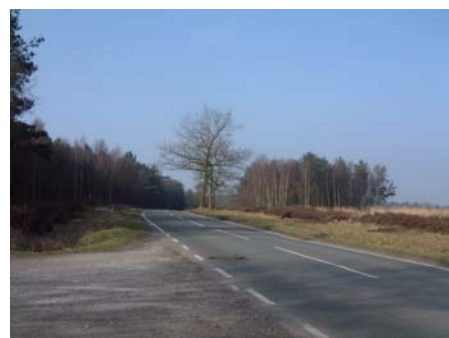
Carriage way edge markings
