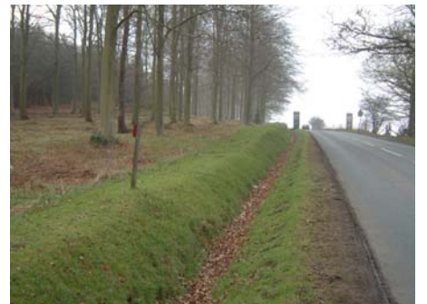
Penkridge Bank Road ditches grassed verges and sett kerbs
