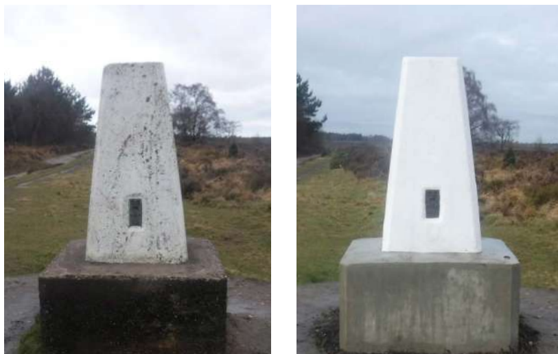
Image: Trig points before and after restoration
