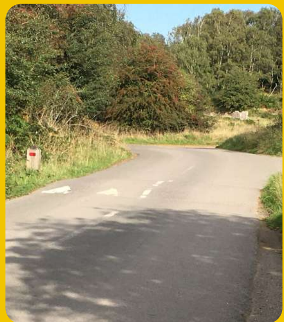
Chase Road traffic calming
