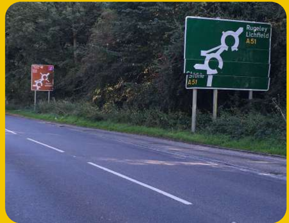
Signage Wolseley Bridge
