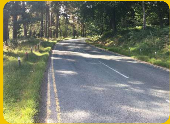
Timber posts and yellow lining, Birches Valley Road
