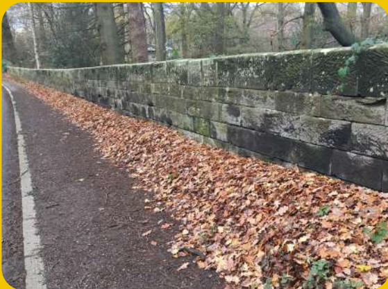
A513 Shugborough Estate boundary: Stone wall, granite road kerb
