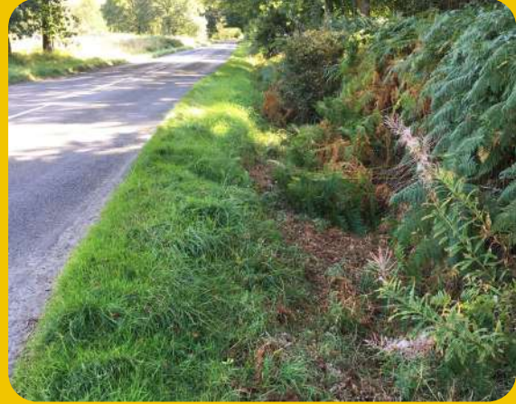
Ditch to discourage vehicular access
