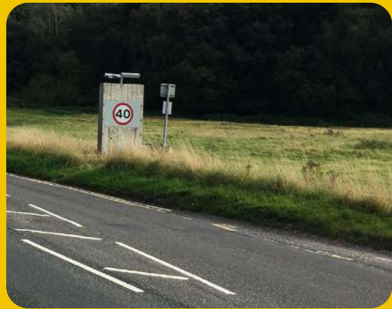
Bund at Milford Common provides visually unobtrusive means of restricting vehicular access
