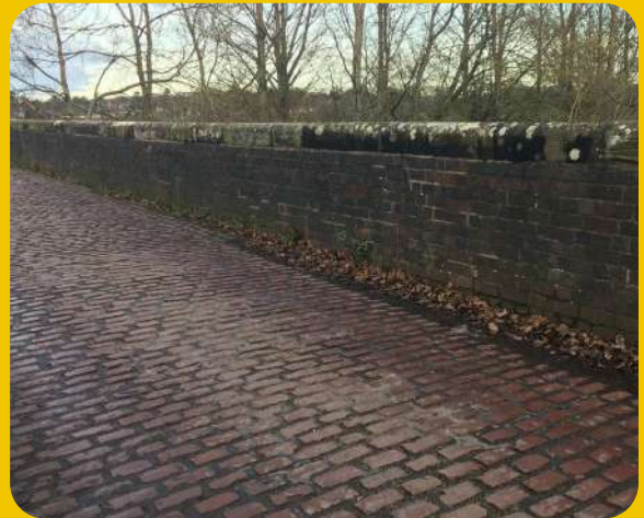
Bridge, Meadow Lane, Little Haywood – brick and stone detailing
