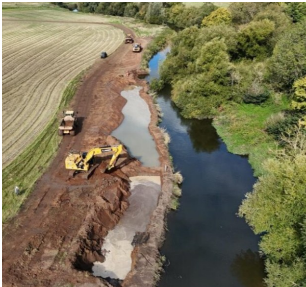
Riverbank re-profiling and river widening
