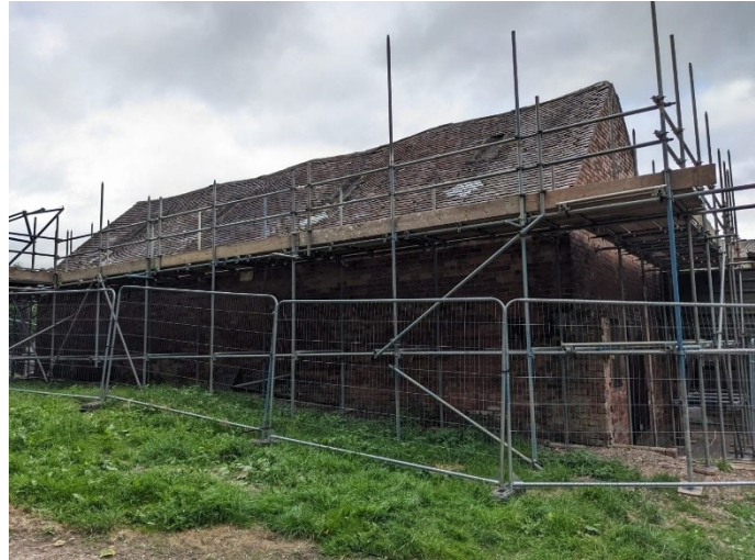
Restoration of historic barn (Cockshutt Barn)
