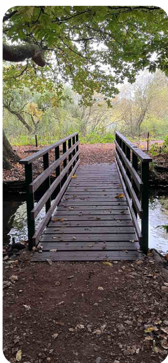
New pedestrian bridge at Wolseley Centre
